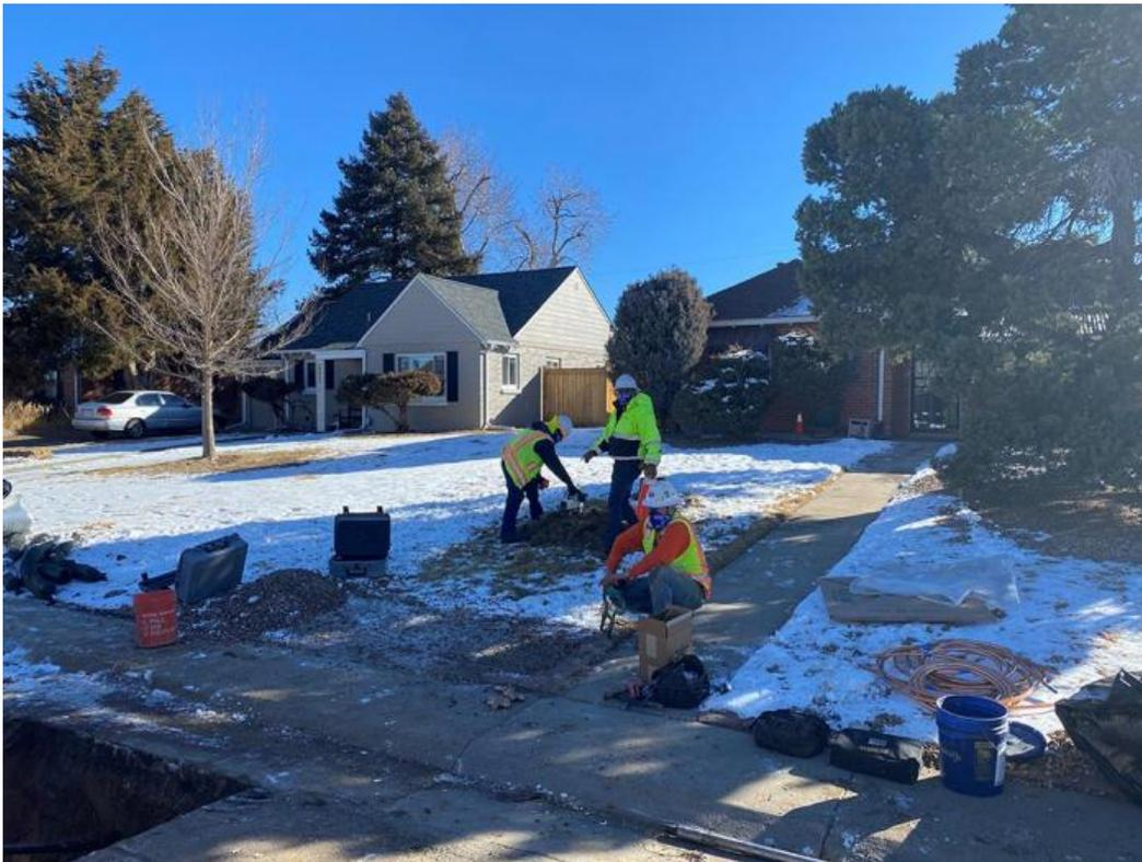
Workers with AGL Construction set to work replacing a lead service line. Photo credit: AGL Construction.
